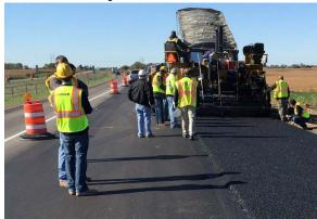
The two different mix designs were produced in sequence with minimal waste. The asphalt mixes were trucked 40 miles on a cool day (55 F at start), and placement temperatures ranged from 235 to 280 F off the trucks. The finished asphalt laid without any tearing, and vibratory rollers produced specified compaction without special effort. The compacted mixes were 1.5" in depth.
