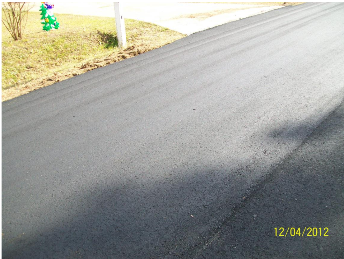
PHOTO 2, Mat after the Rubber Tire Roller.
