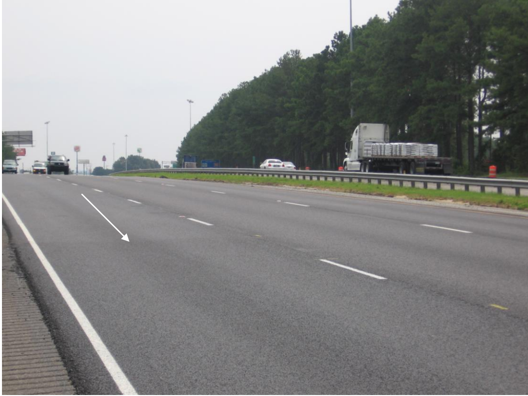
Photo 5 Crumb Rubber/TOR Modified PEM Mixture Joint with Conventional PEM
