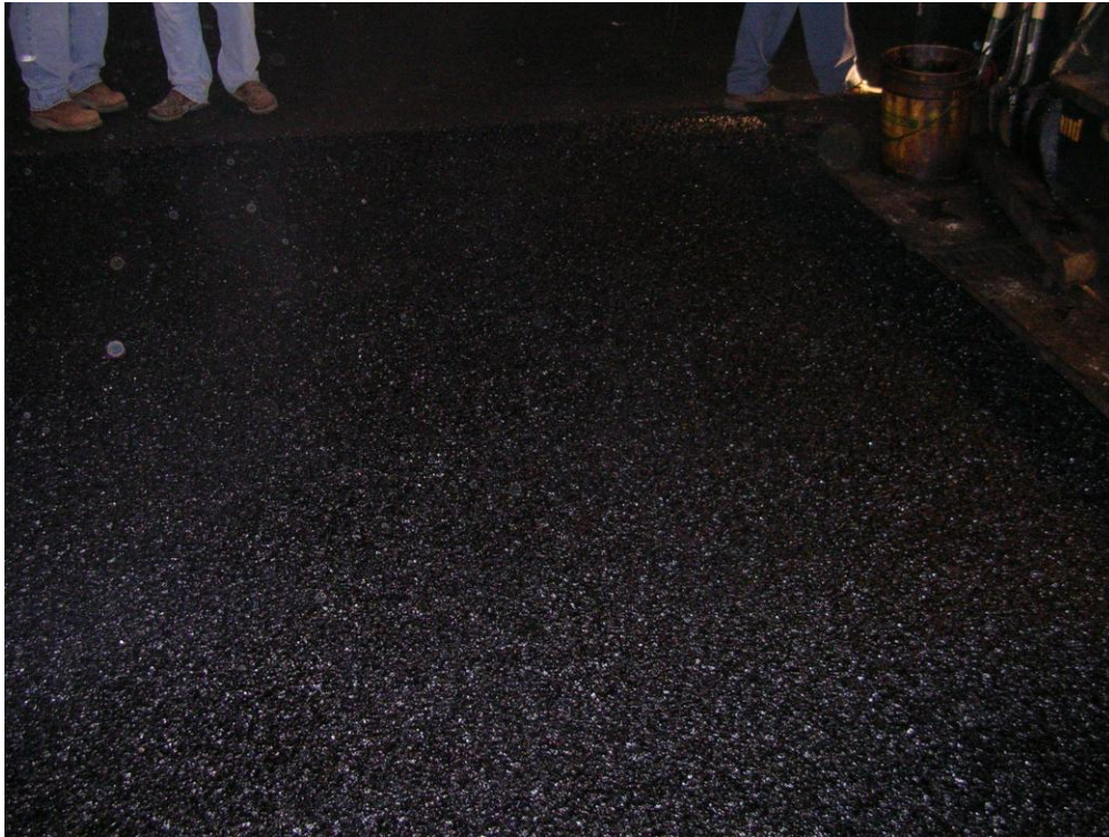
Photo 3 Crumb Rubber/TOR Modified PEM Mixture Behind Paver 8/19/2007
