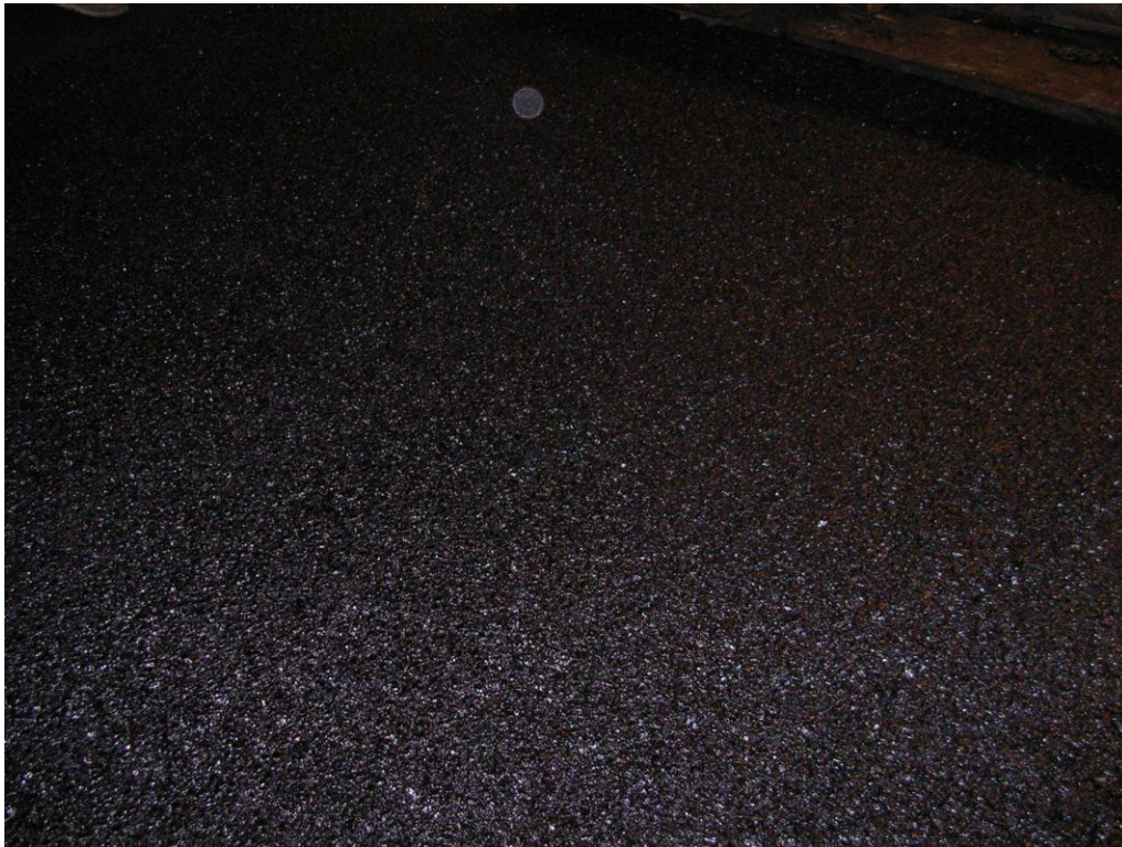
Photo 4 Crumb Rubber/TOR Modified PEM Mixture Behind Paver 8/19/2007
