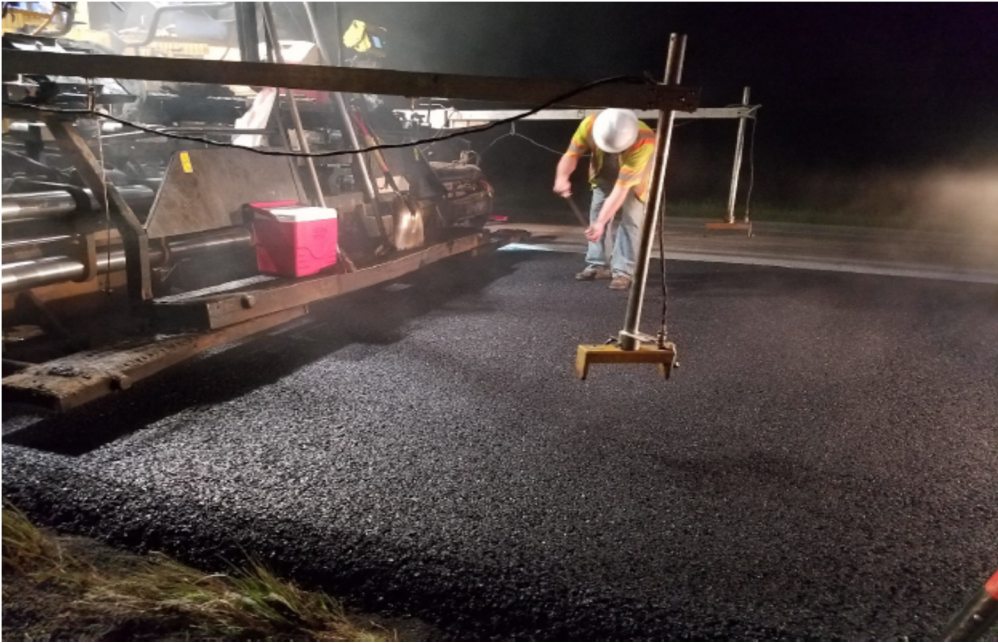
I35 MAINLINE SMA PAVING
