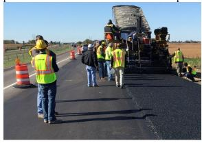
The two different mix designs were produced in sequence with minimal waste. The asphalt mixes were trucked 40 miles on a cool day (55 F at start), and placement temperatures ranged from 235 to 280 F off the trucks. The finished asphalt laid without any tearing, and vibratory rollers produced
