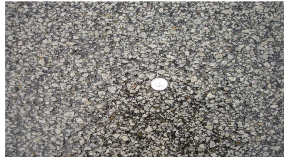
ACCESS ROAD SURFACE CONDITION, 2017
