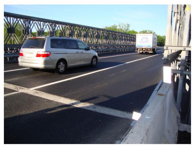
Figure A-12. NJ DOT Bridge Deck Water-proofing Surface Course (BDWSC) on I-80 Bridge (Bennert)
