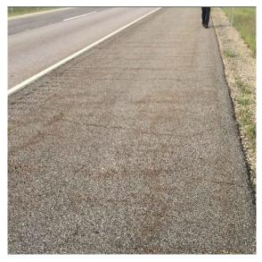
Figure 4-6. Picture from I-88 at mile post 65.9-High ABR rubber modified asphalt (RMA) mix (EB shoulder and mainline)
