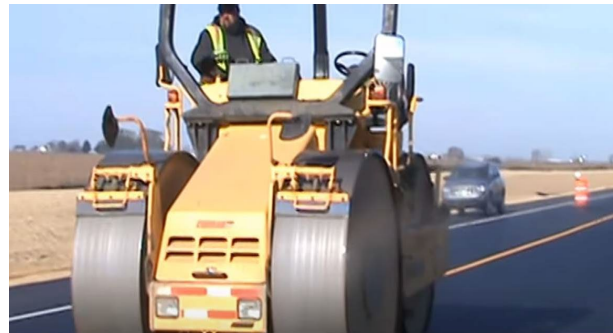
Figure 1: Compaction on I-88, Fall, 2015
